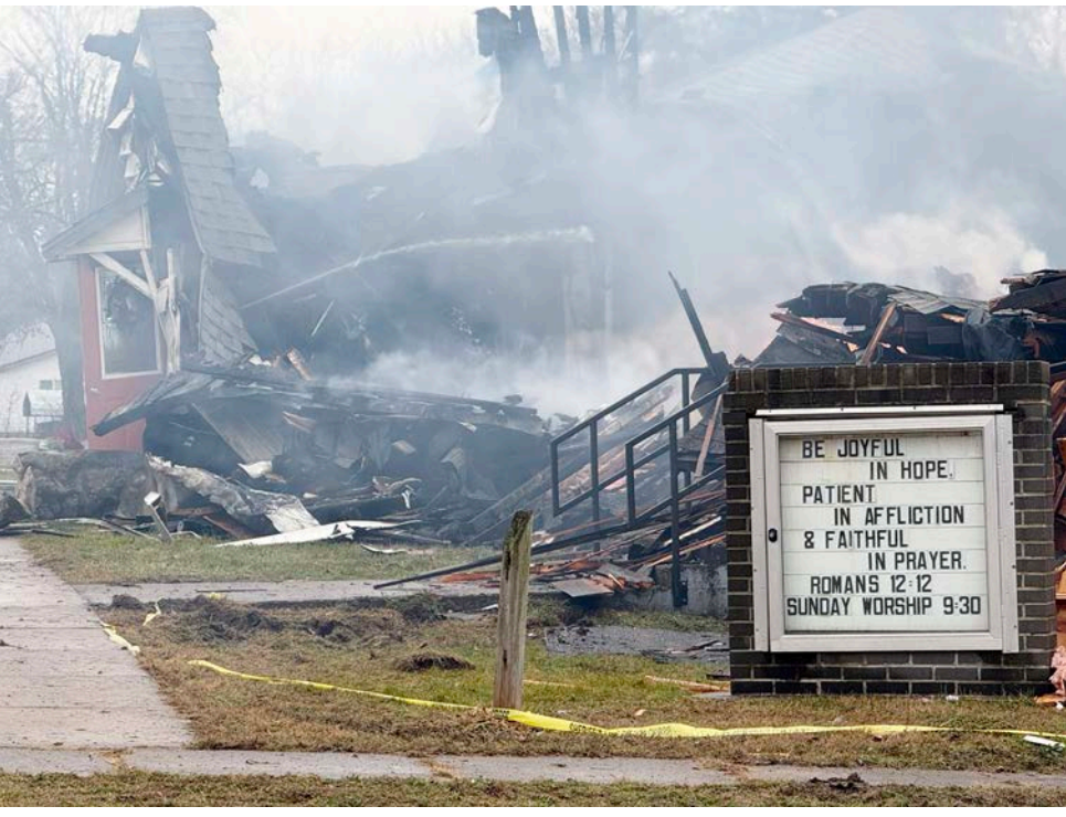
January 2, 2025 edition - Firefighters worked to tamp down rekindled hot spots in the smoldering remains of the Colony Community Church, which caught fire the night before.
