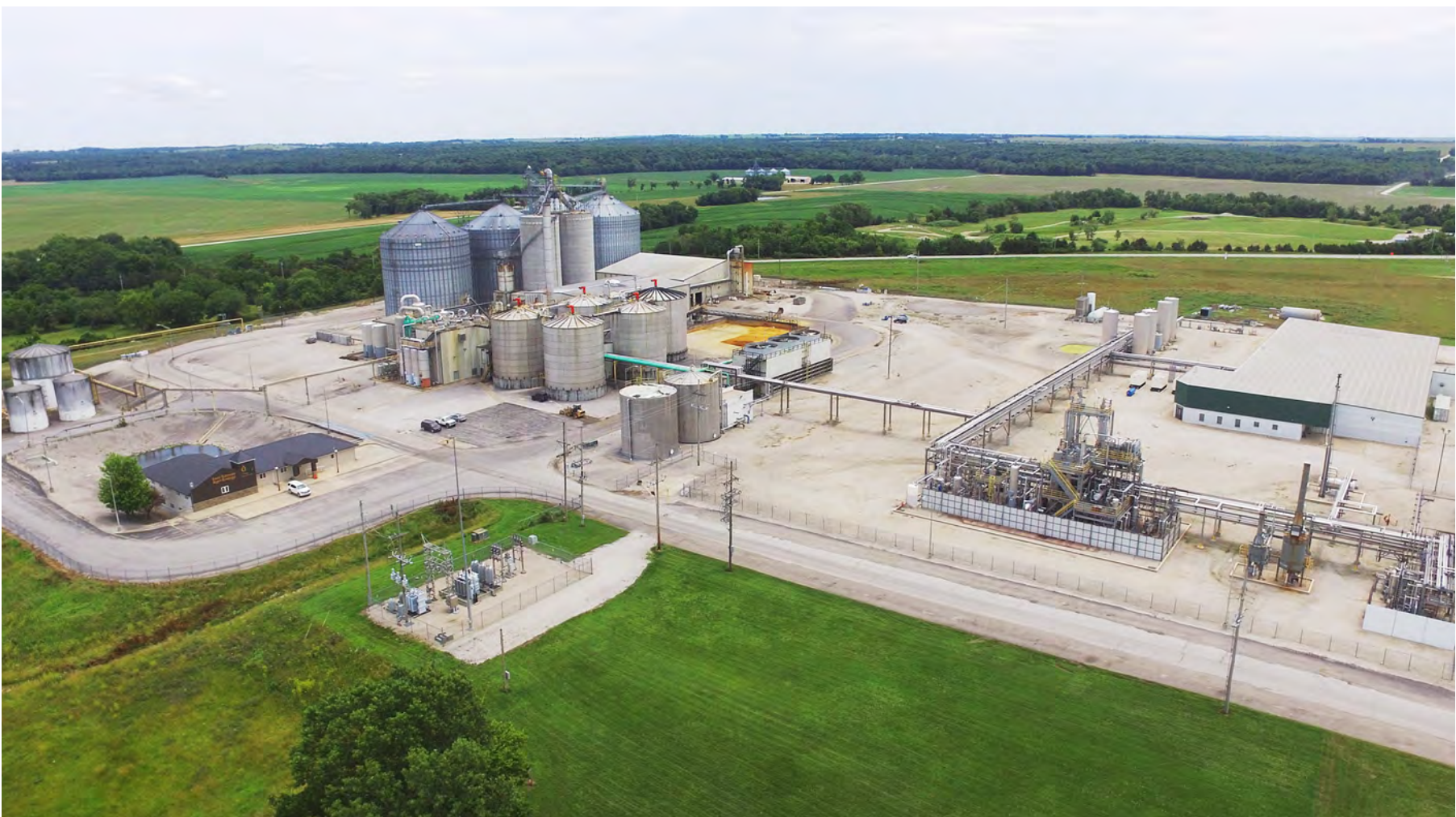
EKAE's campus expanded from its original size with the addition of a renewable diesel production facility at right and additional grain storage bins constructed along its U.S. Highway 169 frontage.
