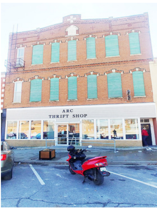
THE ANDERSON COUNTY REVIEW 1-31-2023 / DANE HICKS Garnett's Arc Thrift Shop is looking for location options with word the local Delphian Lodge hopes to sell the building where Arc is a tenant.
