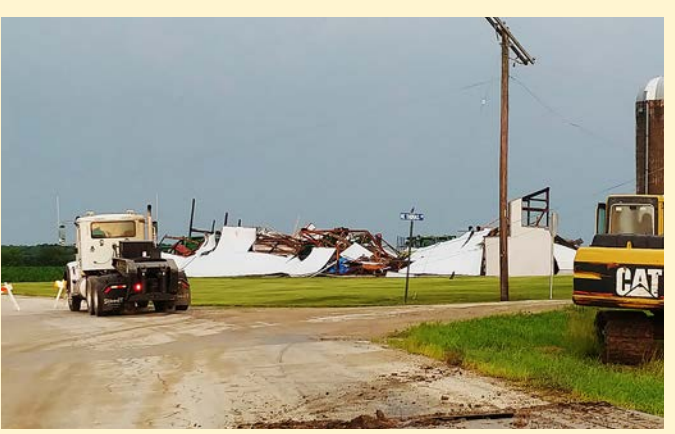
Road (top right) lost a portion of its roof, a huge tree uprooted a section of sidewalk on East Fourth Avenue, and an equipment shed at the Joe Peine residence near Greeley was destroyed.
