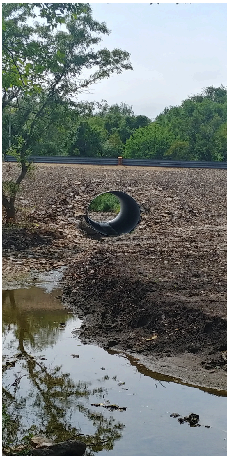
THE ANDERSON COUNTY REVIEW 8-27-2019 / DANE HICKS Repairs have been completed on Lake Garnett Road’s west culvert in time for the upcoming Garnett Grand Prix Revival road car exhibition. The culvert was damaged last month by heavy rains.
