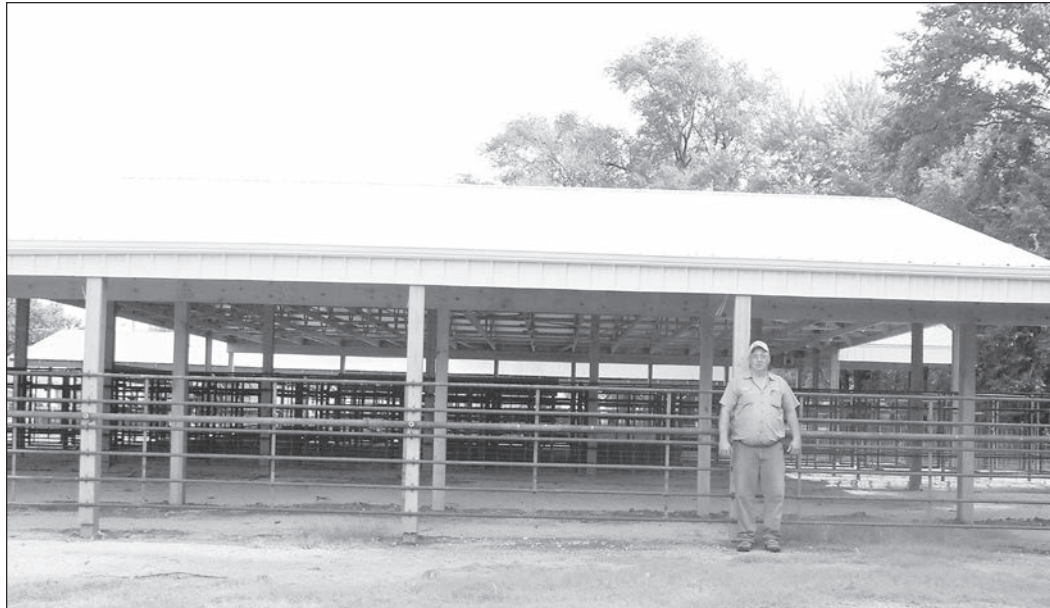
THE ANDERSON COUNTY REVIEW 07-11-2017 / Photo Submitted Doyle Sobba in front of the addition to the fair barn at Richmond. Sobba headed the 20x60 foot addition that was provided by QSI (Quality Structures, Inc.), which will allow much more room for livestock.
