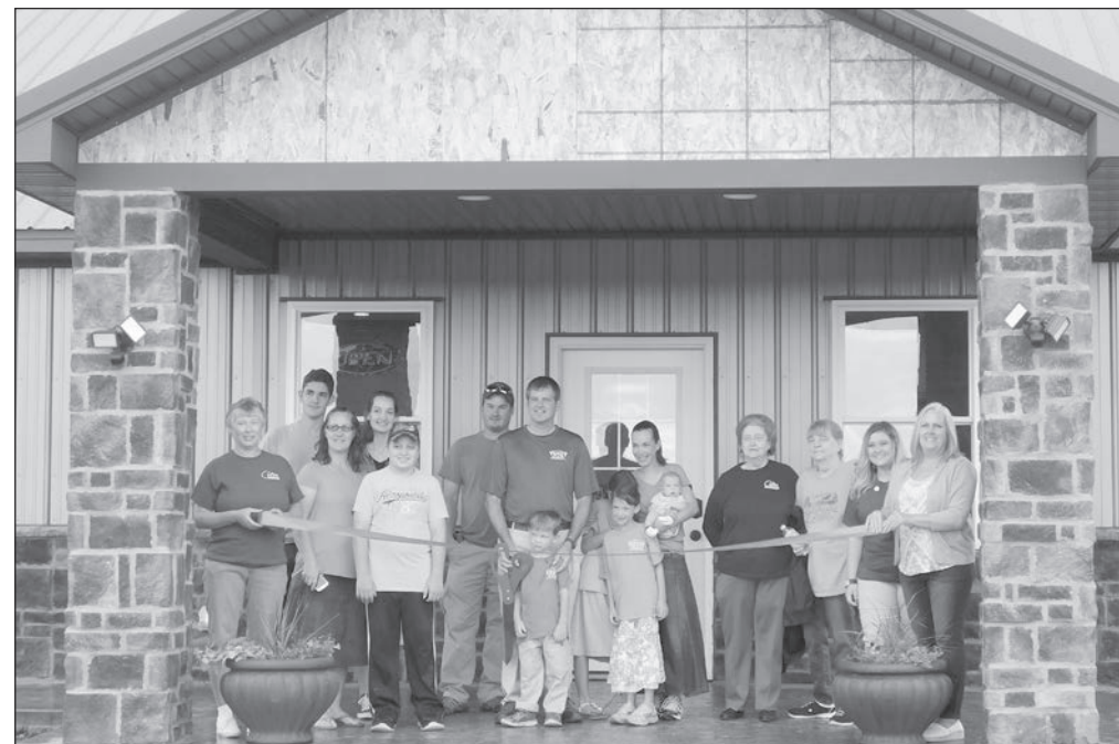
A new operations center has been built for Yutzy Construction of Garnett south of the U.S. 59/169 highway roundabout. Pictured (l-r): Paula Sjolund, Jeremiah Riehl, Becky Riehl, Kathleen Riehl, Nick Stoltzfus (blue), Vernon Yoder, Daniel Yutzy, Miciah Yutzy, Grace Yutzy, Gloria Yutzy, Faye Yutzy, Maciah Yutzy, Twyla Duryea, Penny Layton, Desiree Donovan and Sheri Lickteig.
