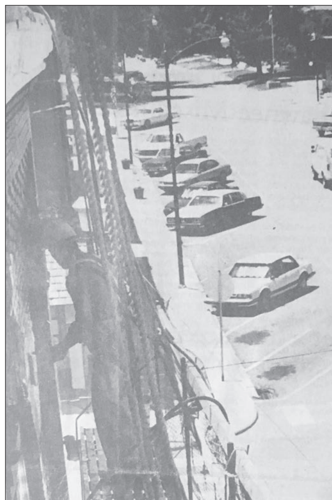
Workers from Fort Scott complete a portion of the tuck pointing job on Garnett State Savings Bank in 1996 against a background of West Fifth Avenue.
