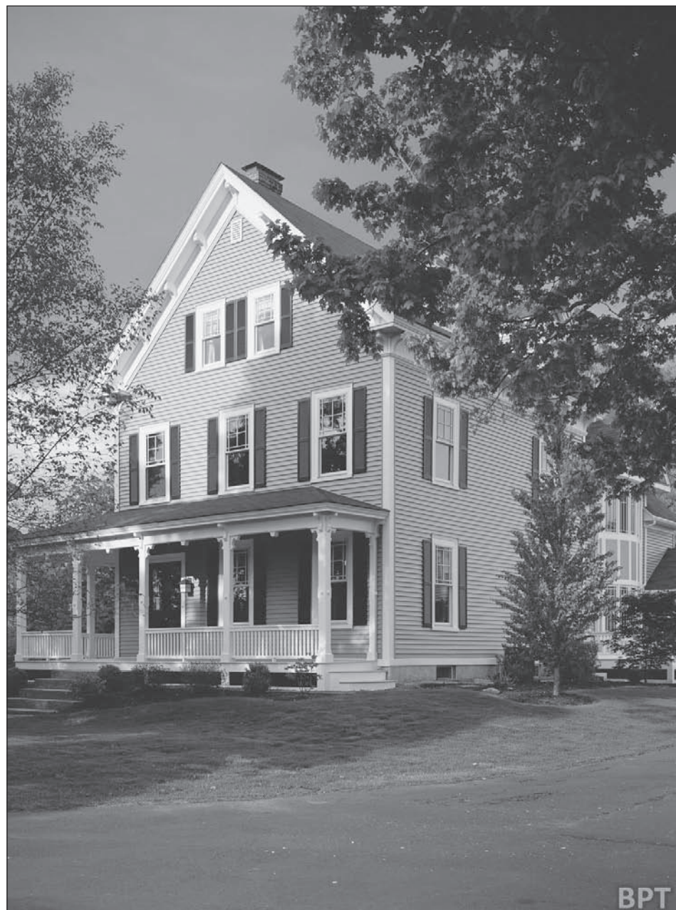
Now's the time to inspect your home's windows and doors to make sure you're getting the most energy efficiency. Courtesy of Brandpoint Content
