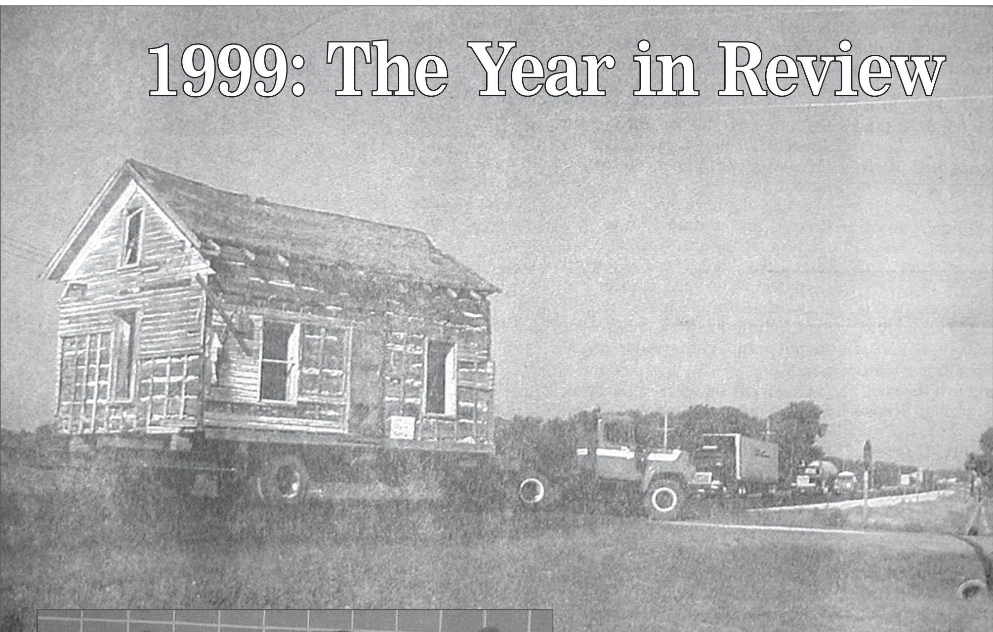
The 1856 Valentine Gerth cabin, home of Anderson County's first white settler, slowly makes a turn from 169 Highway onto Main Street in Greeley July 8, taking the cabin from its original homestead just north of the cemetery on Trego Road to its new foundation near the wagon bridge in Greeley. Efforts to save the cabin began in mid-May.
