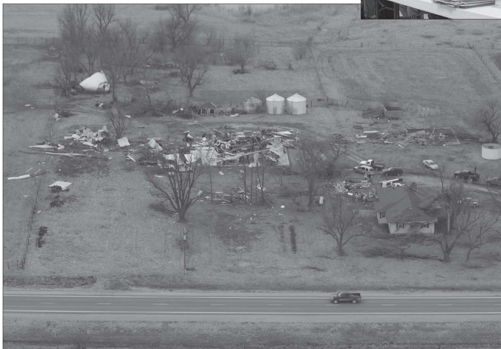
The Howarter property showed the type of damage indicated to many sites in the area after a tornado swept through the county in March. Houses were missing shingles but still standing while outbuildings, vehicles and some equipment were swept from their locations and in some cases hundreds of yards.
