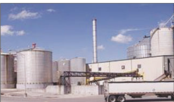
The East Kansas Agri-Energy plant in Garnett is expected to suspend production Oct. 1. Plant officials say the plant may not open until next summer.
