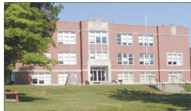
Garnett Elementary Center is scheduled to be demolished in July, but some hope it can still be saved.
